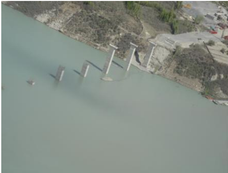
Submerged pillars of an under construction bridge
