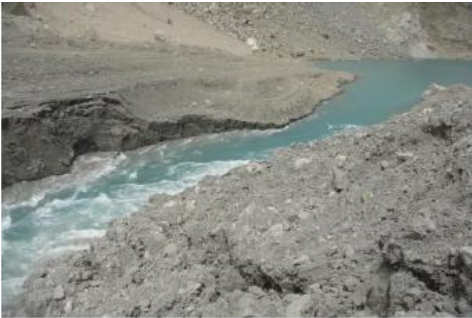
A view of Hunza lake spillway
